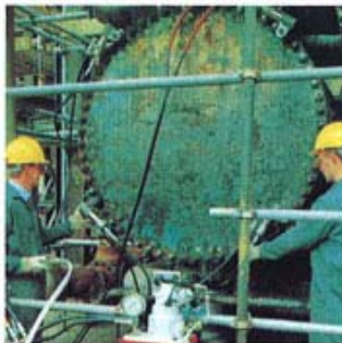
Four wrenches being used simultaneously, powered by one pump.
